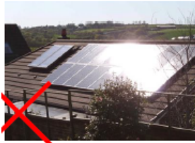
Poorly positioned solar panels
